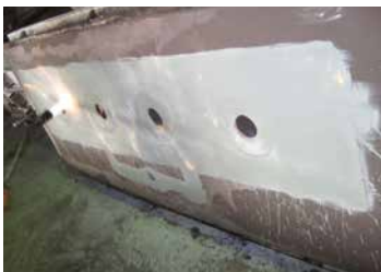
Figure 12: Correct drying of the coating
