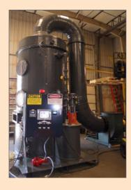
Core/Mold Making Properties - A sand trap installed between the E-A/SO<sub>2</sub> core machine and scrubber is often recommended. This is a very effective way to prevent fine sand particles from entering the scrubber.
